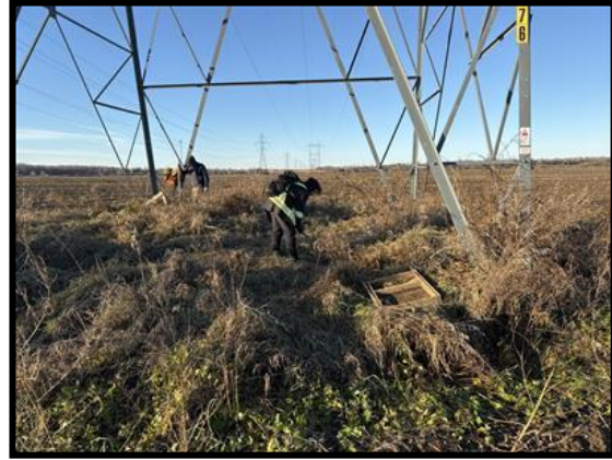
Image 14: Test Pit Survey (November 27, 2024; Facing West)
