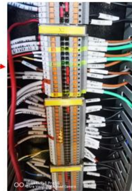
F-STOP signal input: X3:27,X3:37
